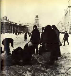
A burst pipe cuts off water supplies. People bring pails to a hastily fixed-up stand-pipe in Nevsky Prospect, the main street
